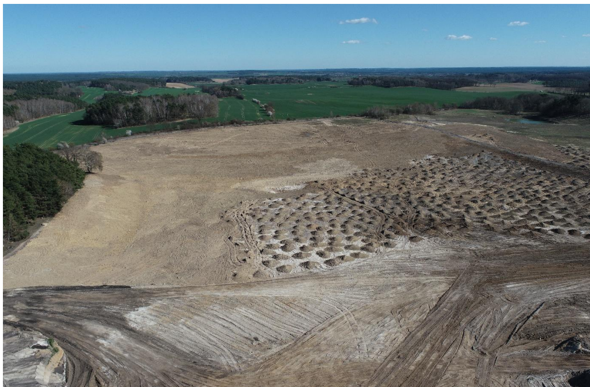
Figure 16. SIENIAWA - spreading the humus layer (humus application).
