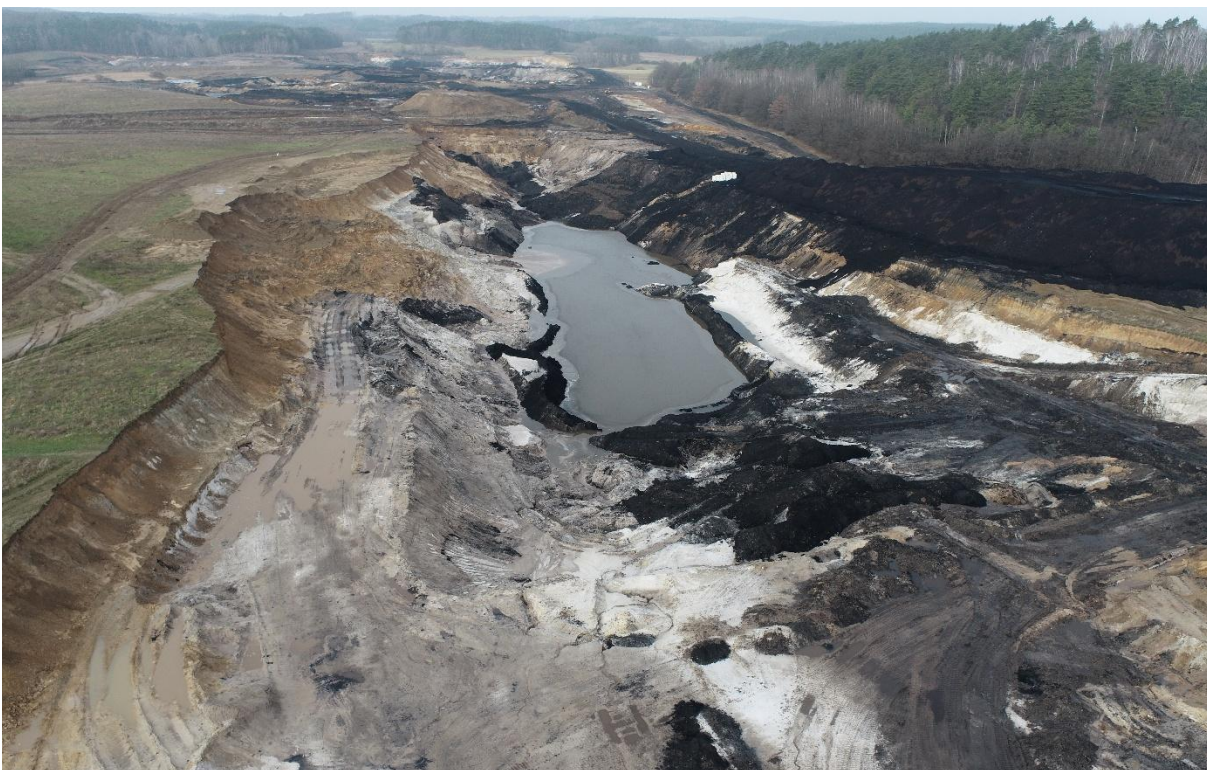
Figure 15. SIENIAWA - reconstruction of the terrain by backfilling the excavations.
