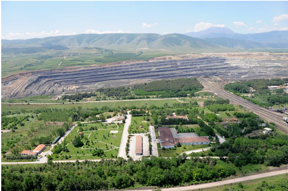
Figure 11. A post-mining area in Western Macedonia (aerial view). The reclamation has been employed in the outside dumping area near Mavropigi mine in Ptolemais mining area.
